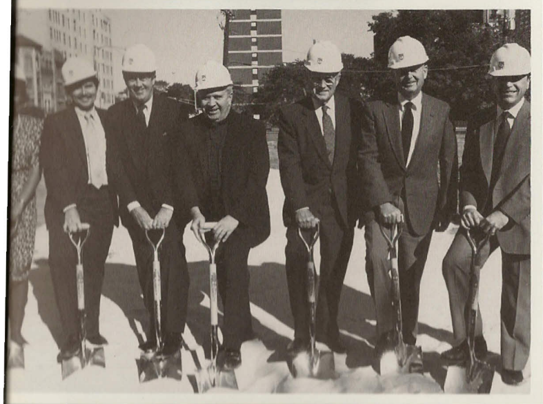
Ground is broken for the Living-Learning Center. Proudly overturning the first shovels of sand at the construction site are student resident Trinean Parker, Alderman David Orr, Executive Vice President Ronald Walker, President Baumhart,
